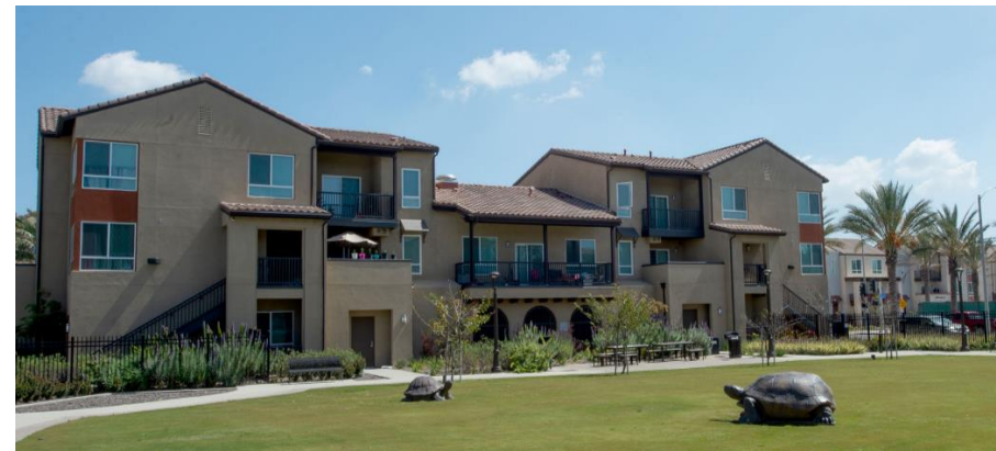
The Jordan Downs revitalization in Los Angeles uses a RAD-Section 18 Blend
